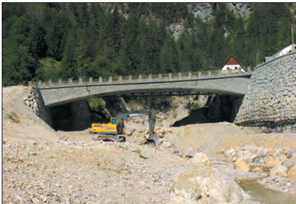
Figure 6: A view of a new reinforced concrete road bridge in Gorenji Log on September 9, 2006 (upstream view, compare the executed bridge with the preliminary design on Figure 5).
