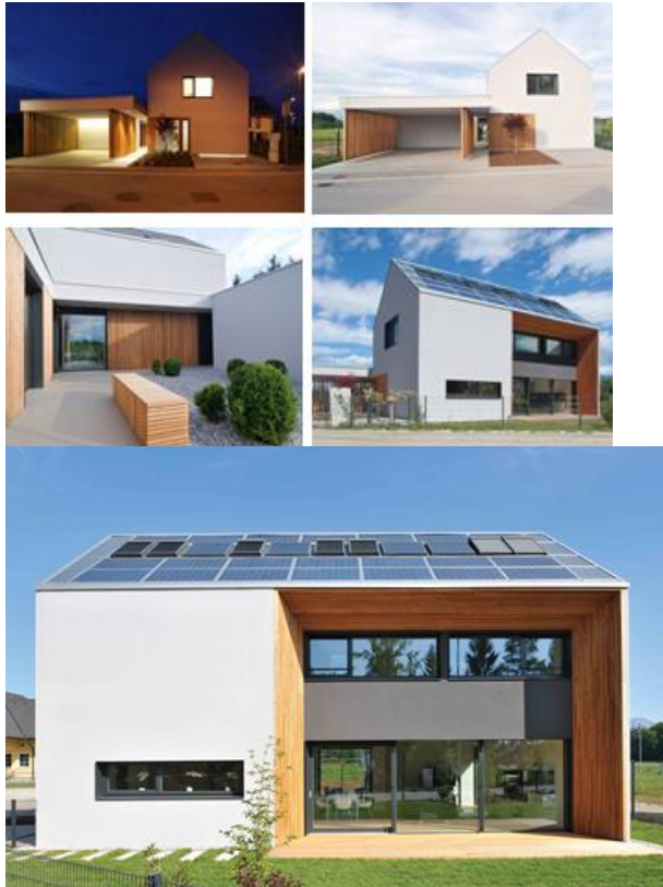
Fig. 7 (a) The house is built entirely of environmentally-friendly materials, which have the biggest impact on the environment in the stage of production. The house includes an photovoltaic power station, solar collectors for hot water, skylights, rainwater gathering for sanitary purposes and watering as well as smart installations, (b) The basic idea in the design was to produce a demonstration dwelling house used for the promotion and relevant explanation about 3 topics energy, indoor climate and environment. Active House is a network for knowledge sharing and demonstration of the feasibility of comfortable buildings in the future.
